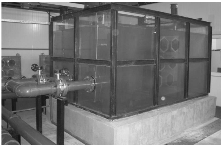
Fig. 7. Photograph 3 of the test system (containment sump strainers)
